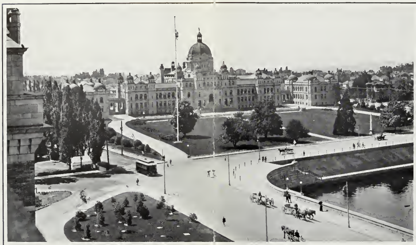
General View of British Columbia Parliament Buildings at Victoria, showing Hassam Pavement in Driveways
